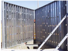
C-Joist supporting marble
