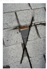
Knock out cut
